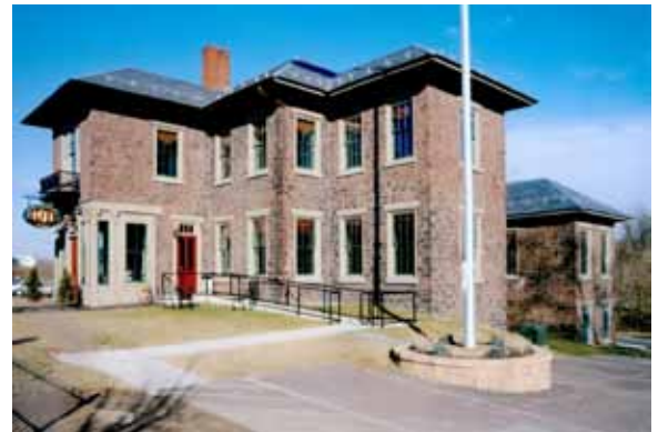
Phoenixville Foundry - Superintendent's Building, Chester County. PHMC Photo Collection.
