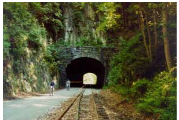
York County Heritage Rail Trail - Howard Tunnel, York County. PHMC Photo Collection.
