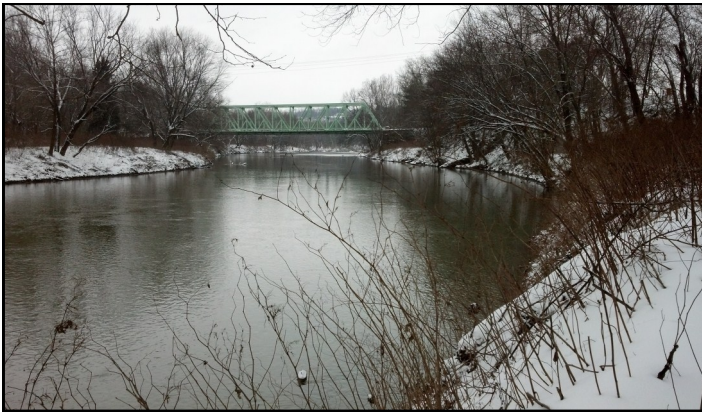
Conemaugh River/Bairdstown Bridge. Source: BCDA
