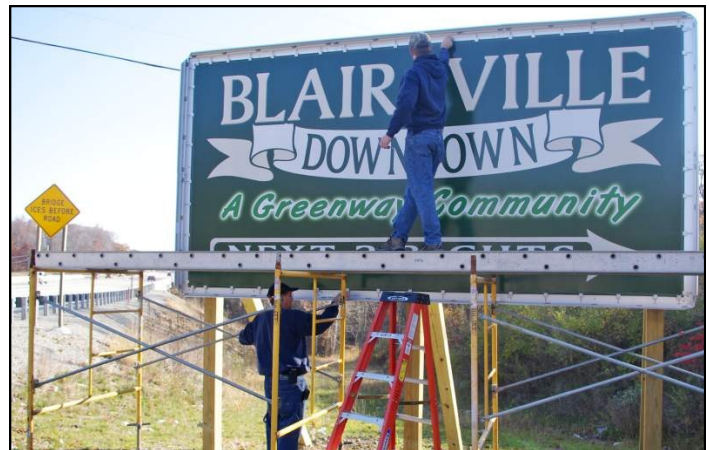
Installing new gateway signage along Route 22. Source: www.triblive.com
