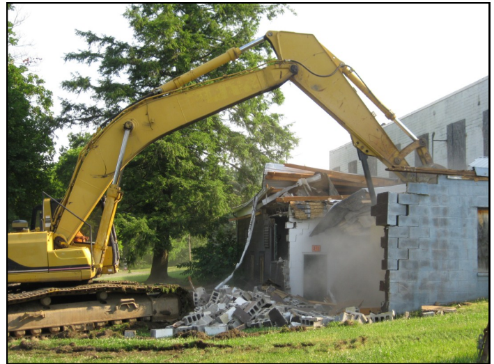
Demolition of vacant building on North Liberty Street. Blairsville, PA: Source: BCDA
